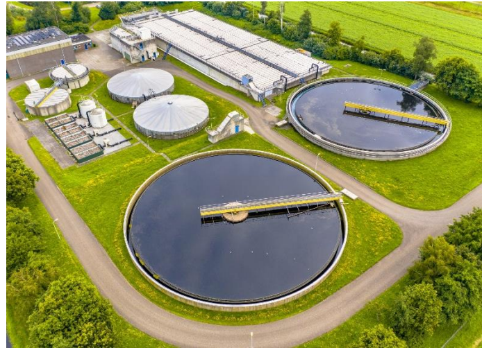
Wastewater treatment plant (Capacity is 2-3 mean daily discharge)
